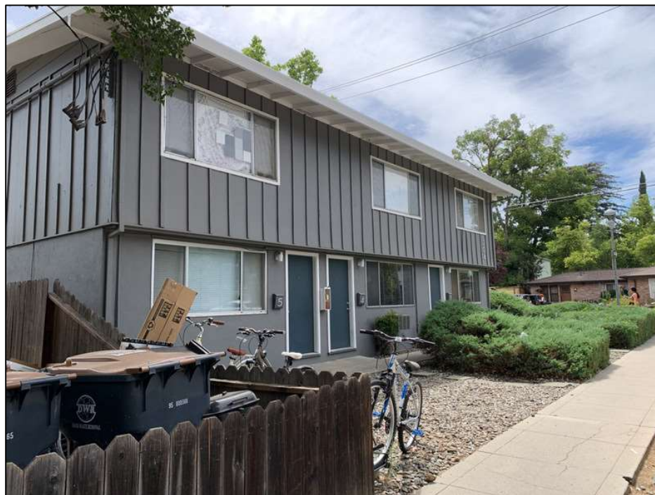
P5b. Description of Photo: West façade, looking south, ESA 2022
