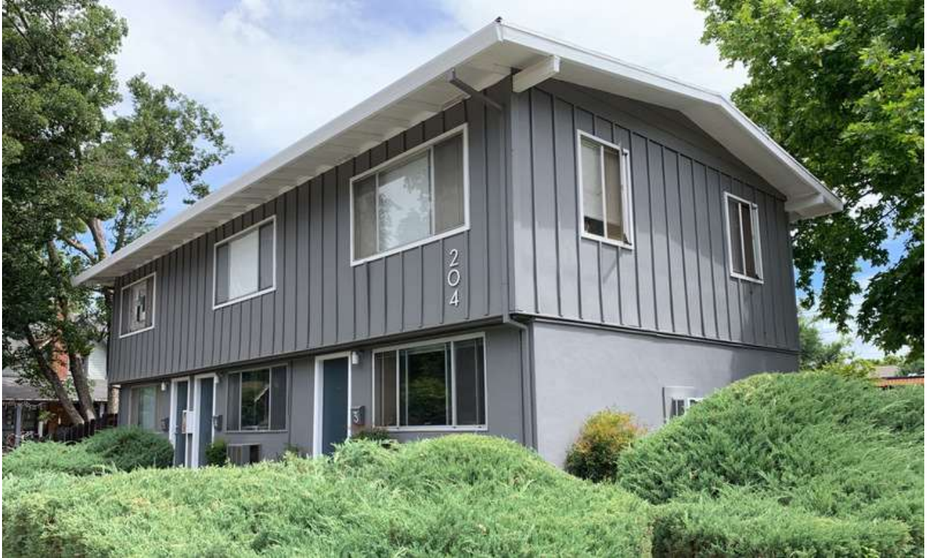
Westernmost building, west and south facades, ESA 2022
